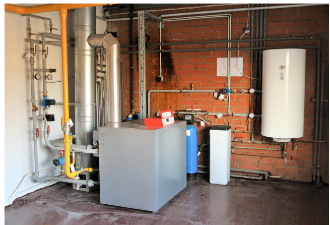
Typical HVAC Hydronic Boiler Systems
