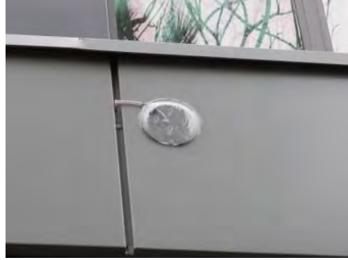
Figure 3.6 Exterior pressure tap with cover to protect the end of the tube from water.
