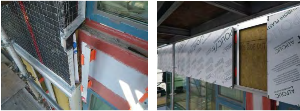
Figure 4.3 Stucco (left) and metal panels (right) are installed over the insulation.
