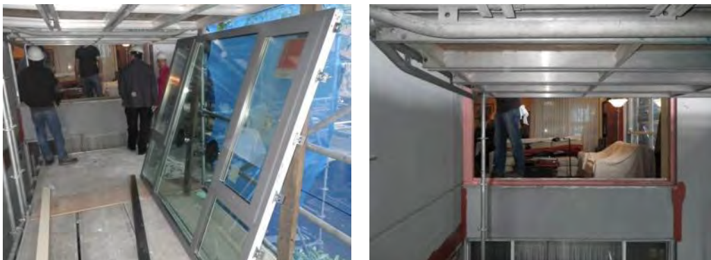
Figure 4.4 Installing the new triple glazed fiberglass frame windows.
