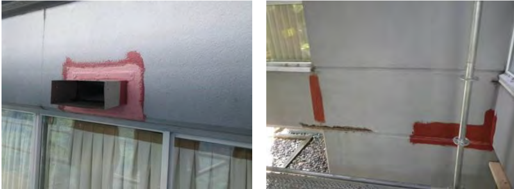
Figure 4.6 Airtight detailing around vents (left) and partial installation of a liquid applied barrier over concrete cracks and cold joints (right).
