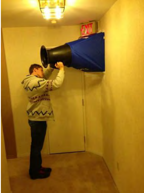
Figure 5.3 Balometer being used to measure airflow supply rate to a corridor from the MAU.
