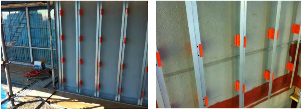
Figure 4.1 Fibreglass clips and z-girts are screwed to the exterior concrete walls.
