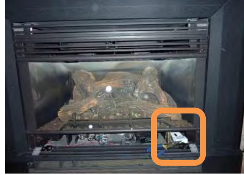
Figure 3.19 Typical SMT-A2 installed under a fireplace. A temperature sensor is installed near the pilot light to provide an indicator of fireplace use.
