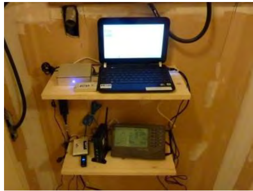
Figure 3.8 One of two BiGs (laptop) located in an electrical closet to communicate with data acquisition units distributed throughout building. The weather station console and communications equipment (to access the internet) are also visible on the lower shelf.
