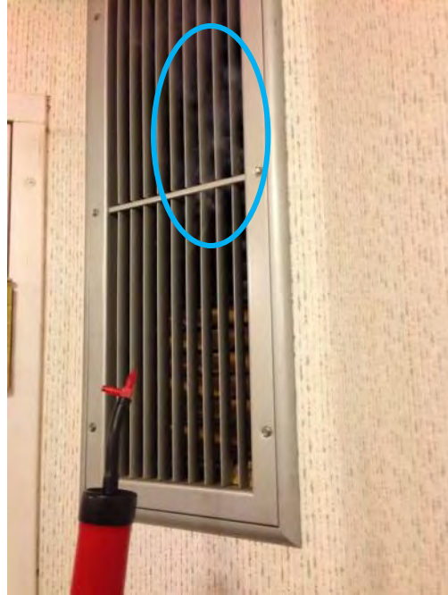
Figure 5.4 A smoke pencil being used to check the airflow direction out of the MAU grille with the MAU off showing smoke flowing back into the MAU duct.
