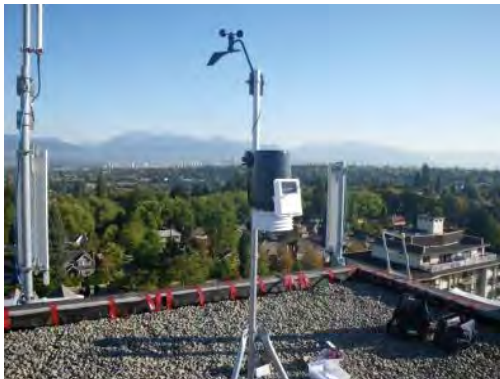
Figure 3.7 Weather station installed on roof of retrofit building to measure temperature, relative humidity, solar radiation, wind speed and direction, and barometric pressure.
