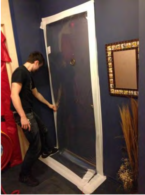
Figure 5.8 Typical suite entrance door sealed with a polyethylene sheet and tape to prevent airflow. By measuring the corridor air leakage with and without each this door sealed, the airflow rate through the door to the suite can be determined.
