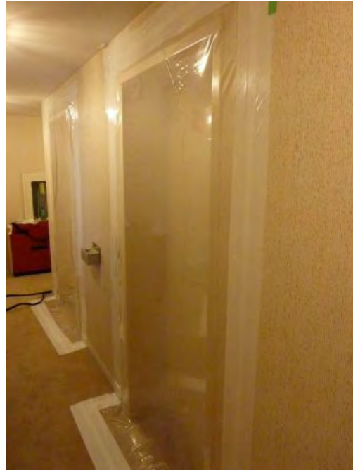
Figure 5.9 Typical sealing of elevator doors to eliminate airflow through the elevator doors to the shaft. A significant amount of corridor air leakage was found to be to the elevator shaft through these doors.
