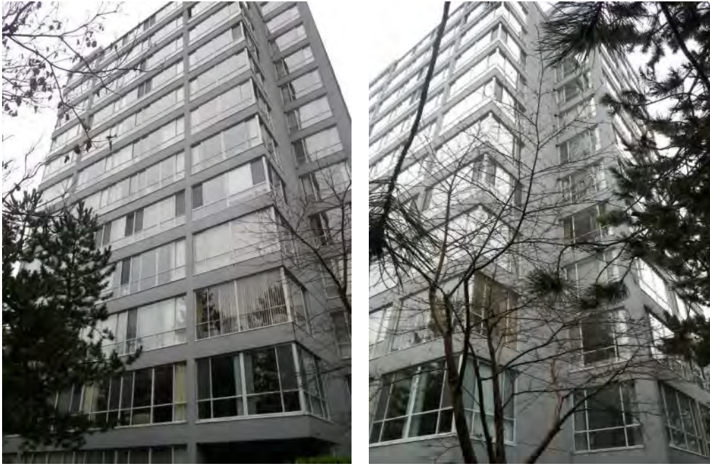
Figure 2.1 North elevation (left) and partial north and west elevations (right).
