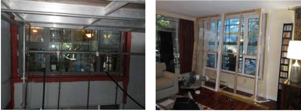
Figure 4.5 Testing the new windows for water penetration resistance.
