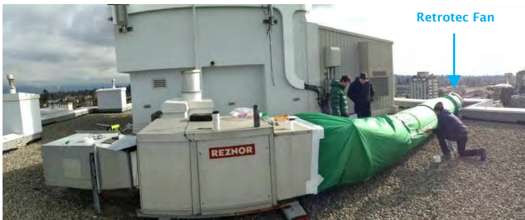
Figure 5.2 Custom made MAU testing apparatus with green flex-duct to attach Retrotec fan to the MAU intake.
