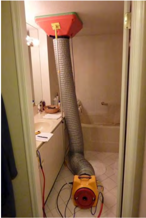
Figure 5.1 Retrotec DucTester being used to test a bathroom fan.
