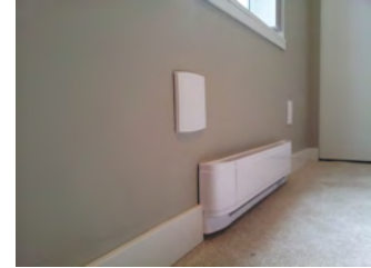
A3 installed in living space
