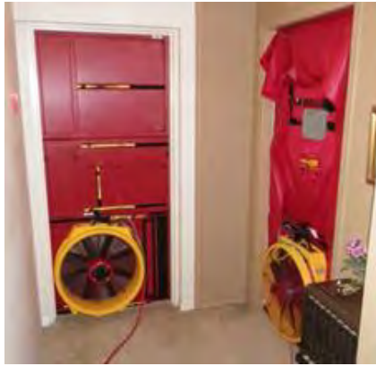
Figure 5.6 Two fan-doors used for airtightness testing. The soft-door with fan installed in the entrance door of a test suite (right door) was used for the test zones as they are more airtight than the hard door units (left door) which were used for the pressure equalized zones where airtightness of the door fan is not as important. Tape was used to seal around the door when necessary.
