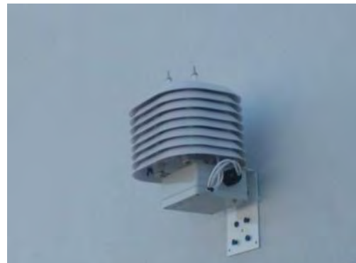
Figure 3.4 SMT-A3 unit installed in a waterproof enclosure for use outside. The SMT-A3 unit is contained in the box on the bottom, and the temperature, relative humidity, and CO 2 sensors are installed within the shroud on top of the box.
