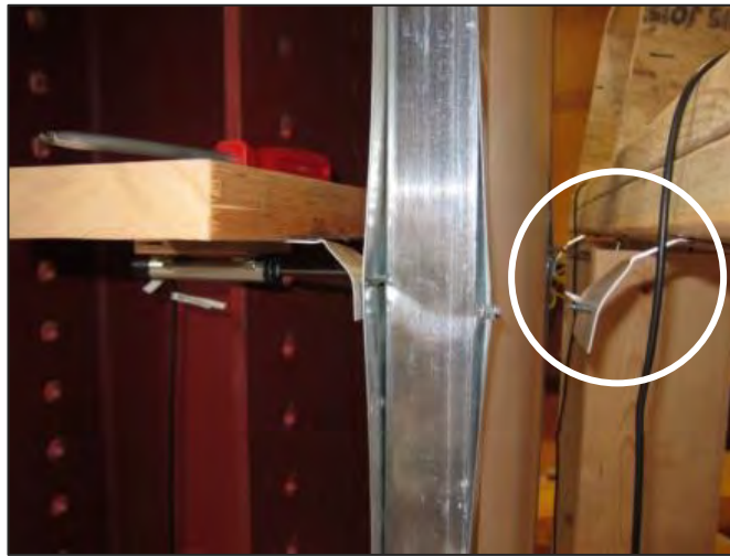
Figure 34 Failure mode of Wall 3
