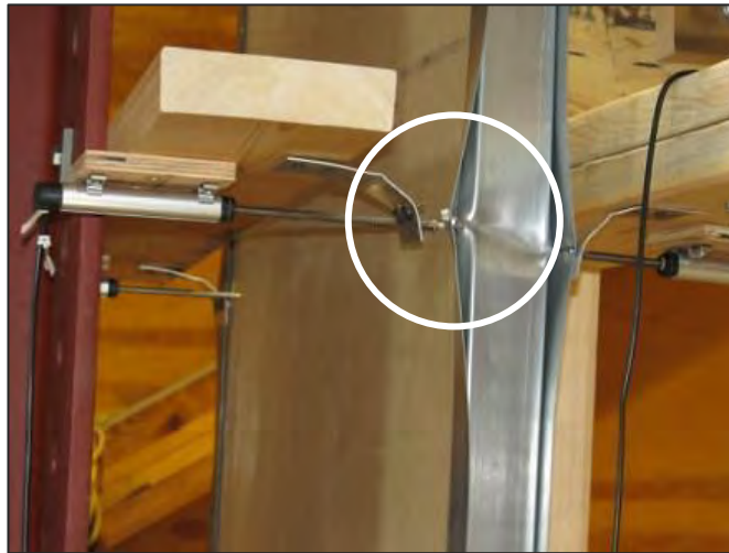
Figure 32 Failure mode of Wall 2
