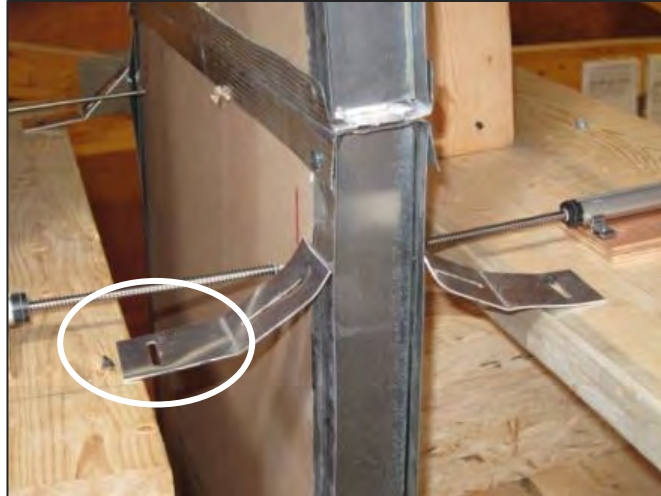
Figure 40 Failure mode of Wall 5
