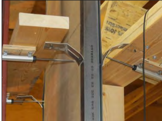
Figure 38 Failure mode of Wall 4
