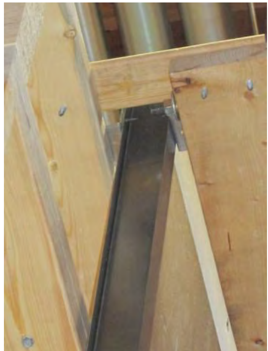
b) Connection at top of wall assembly
