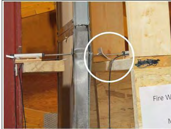
Figure 30 Failure mode of Wall 1
