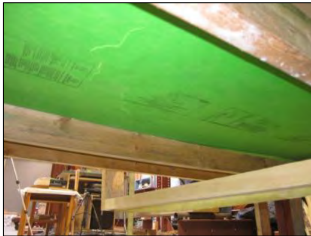
Figure 17 Bottom panel face damage
