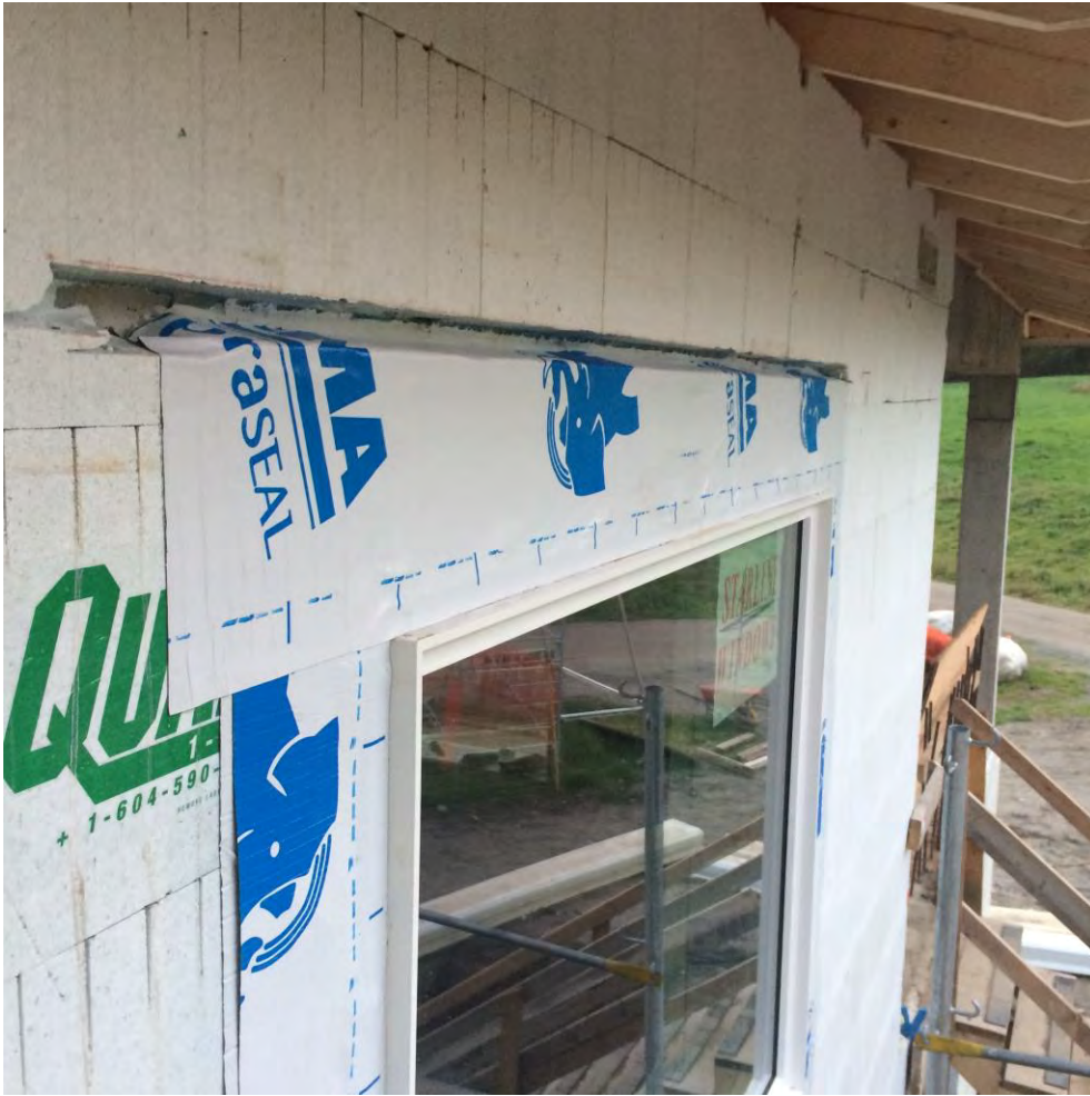
Figure II.7 Module 3 reglet above window head. Note that SAM is sealed to concrete core of ICF.
