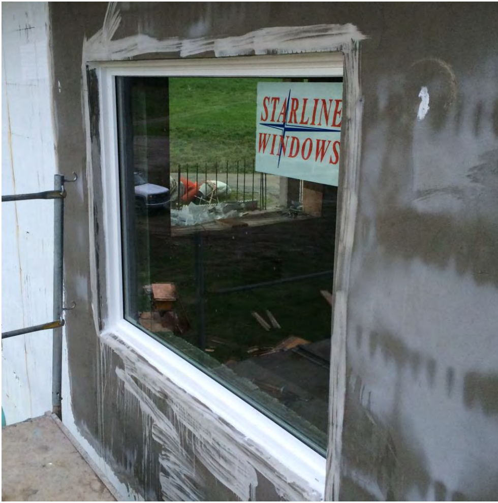
Figure II.4 Window installed in Module 2 rough opening, sealed to EIFS basecoat.
