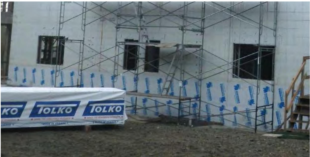
Fig. 4.2.1 Waterproofing membrane terminating on exterior face of ICF foam, with leading edge fully adhered to ICF foam.
