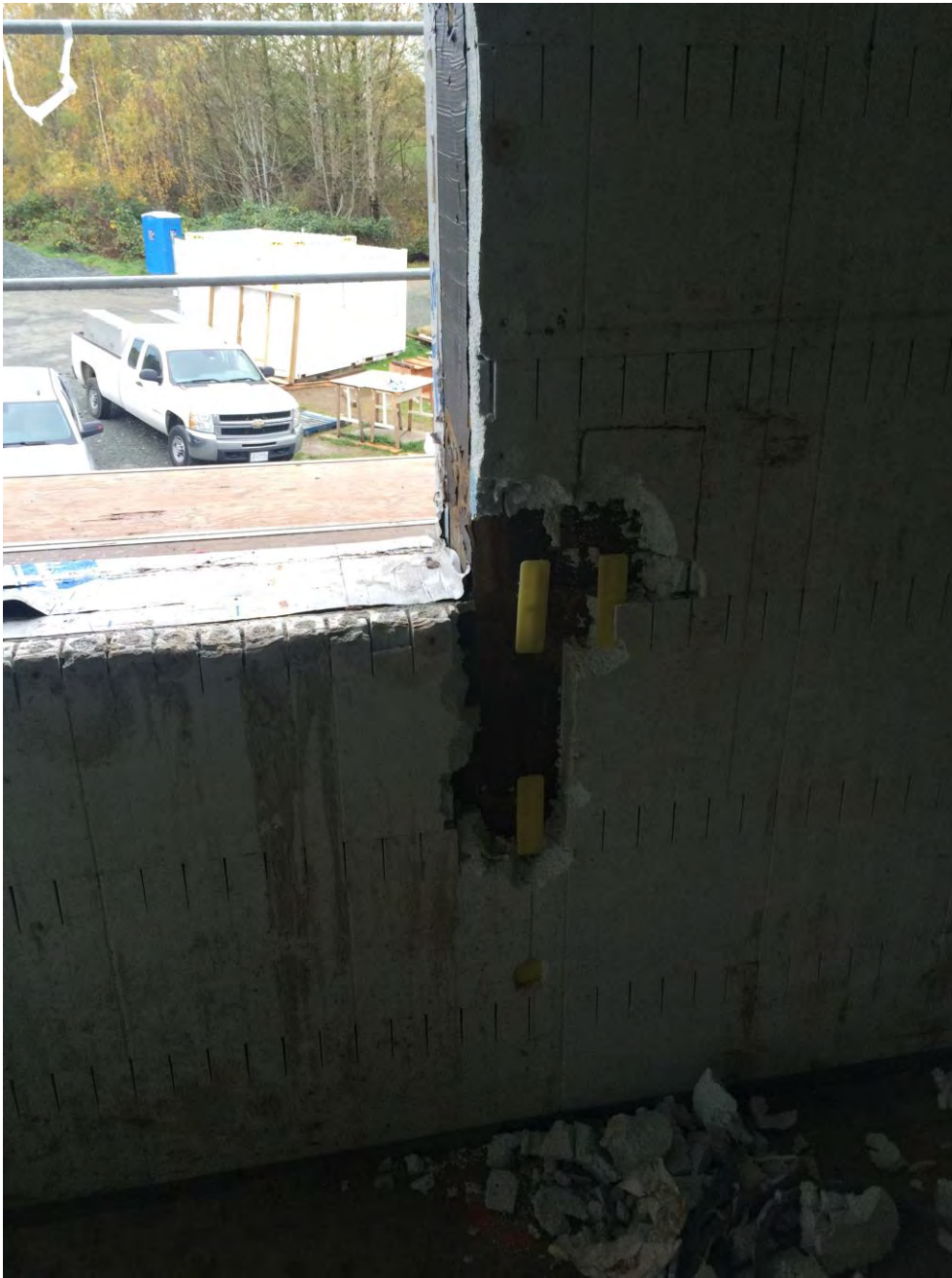
Figure II.8 Module 3 leakage location, below sill at corner.
