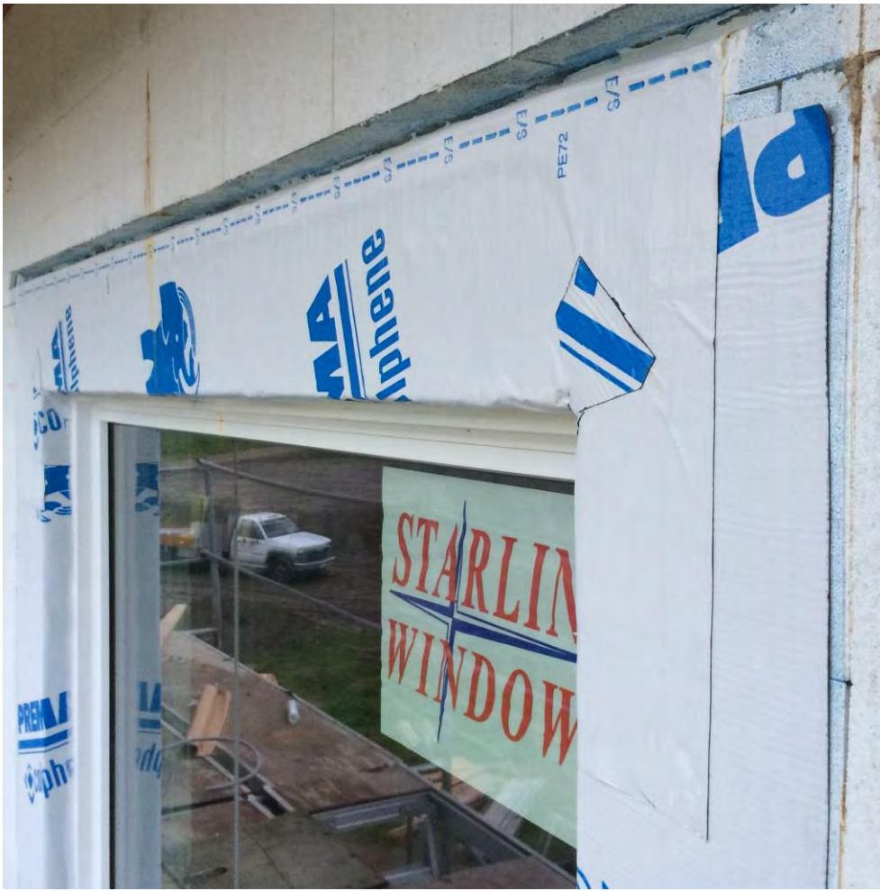
Figure II.1 Exterior of module 1 with window installed. Note reglet above window, sealing window head membrane flashing to concrete core.
