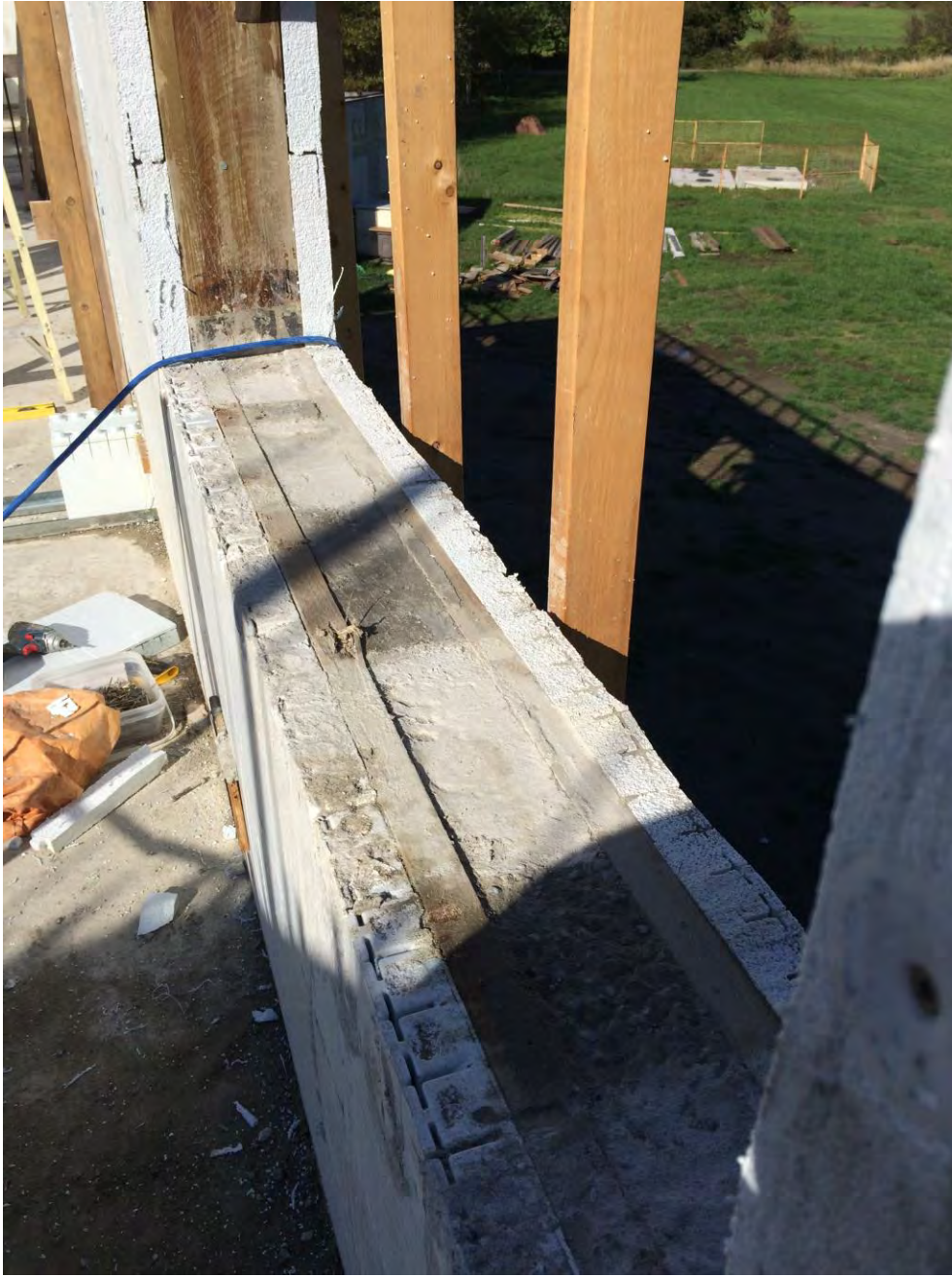
Figure II.3 Module 2 window sill prior to application of EIFS basecoat.
