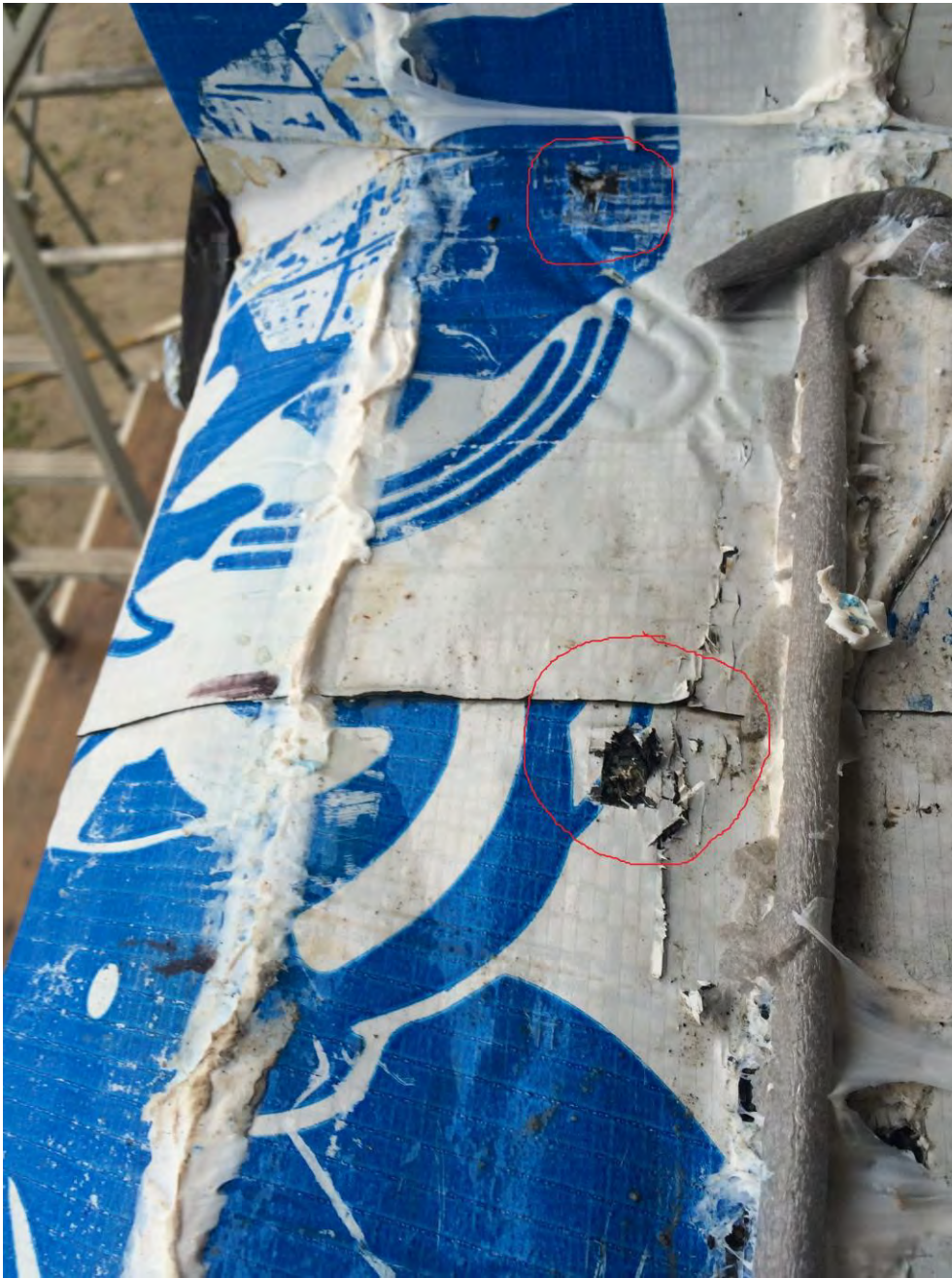
Figure II.2 Module 1 sill flashing after disassembly. Note that hole in membrane corresponds with leakage location.
