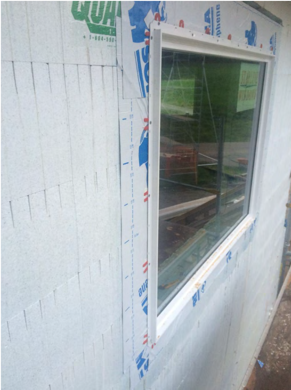
Figure II.6 Module 3 with window installed, prior to sealing exterior of head and jamb flanges with SAM.
