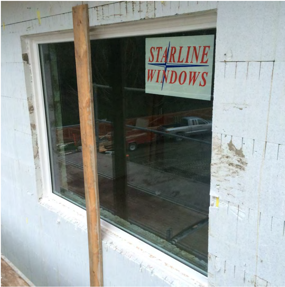
Figure II.9 Module 4 installation. Note that no membrane was provided around window rough opening, seals were all directly between window frame and ICF concrete core.
