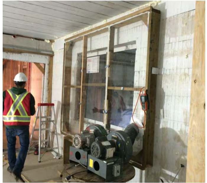
Fig. 3.2.4 Transparent pressure chamber installed on interior face of sample .
