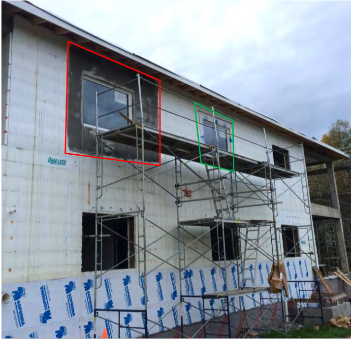
Fig. 3.2.1 Module 2 EIFS Basecoat (outlined in red) and Module 1 Internal Buck with SAM Flashing (outlined in green) on Northwest façade of test building.
