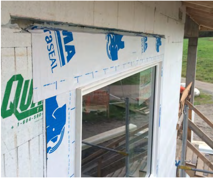
Fig. 3.1.5 Reglet cut into EPS, sealed to concrete, and sloped at 15 degrees to facilitate water shedding and drainage.
