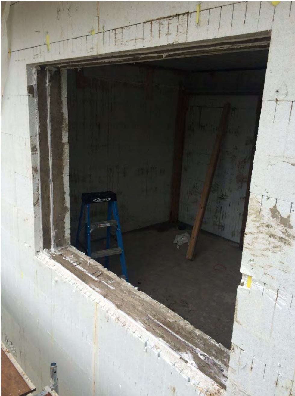
Figure II.11 Module 4 after disassembly, photo taken from exterior scaffolding looking into the building.
