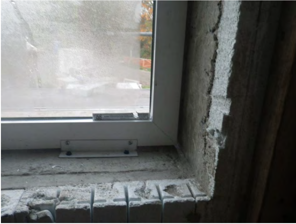
Figure II.10 Corner of window sill, prior to application of backer rod and sealant. Note that window frame was sealed to concrete ICF core and window clips were bedded in caulking prior to fastening to concrete.
