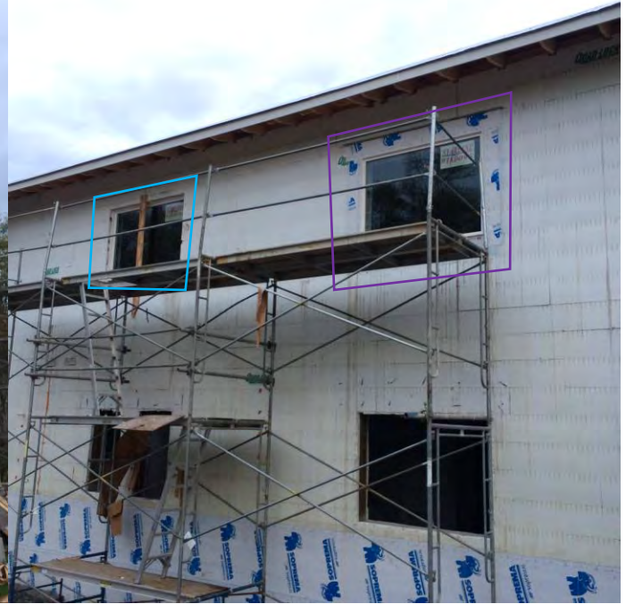
Fig. 3.2.2 Module 4 Direct to Concrete (outlined in blue) and Module 3 External Buck with SAM Flashing (outlined in purple) installed on Southeast face of test building.
