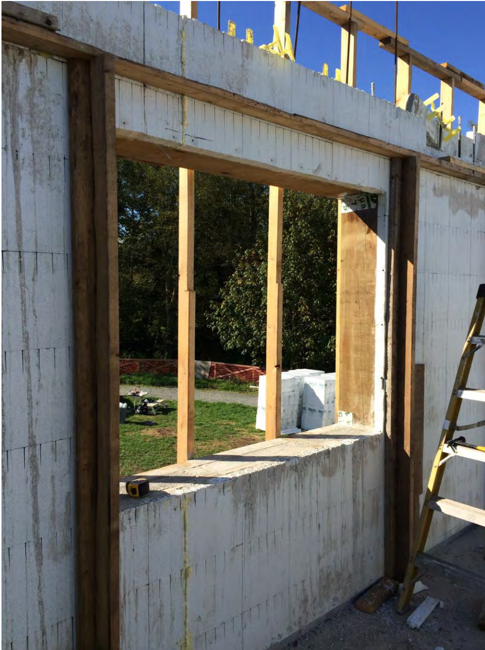
Figure II.5 Module 3 rough opening prior to installation of self-adhered membrane
