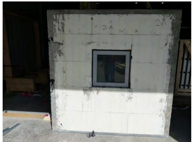
Fig. 1.2.2 Overall exterior view of Module 2A
