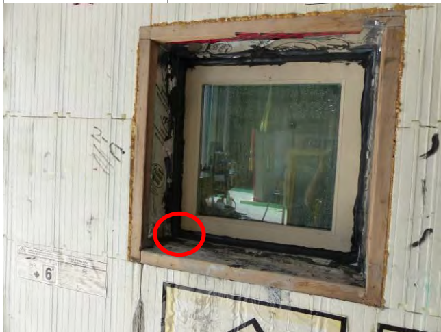
Fig. 4.1.1 Water penetration point P1 for Module 2C at 150 Pa
