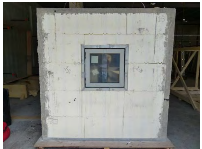
Fig. 1.2.2 Overall exterior view of Module 1B
