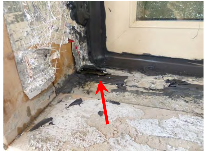
Fig. 4.1.2 Water ingress at lower left-hand corner of window penetrated through the fasteners
