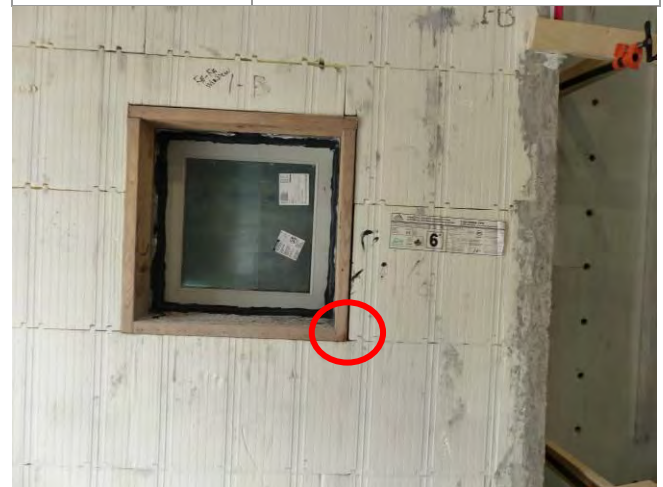
Fig. 4.3.1 Water penetration point P1 for Module 1B at 700 Pa
