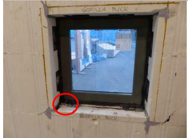
Fig. 4.2.2 Water penetration point P1 for Gorilla Buck Module at 300 Pa
