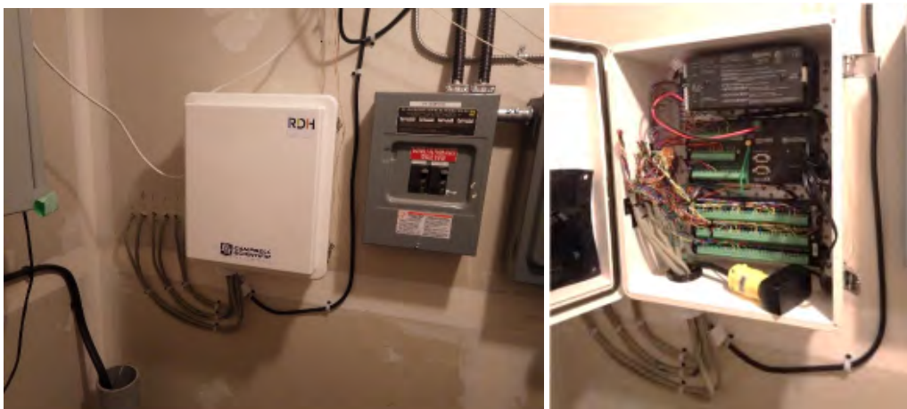
Figure 3-8 – Campbell Scientific CR1000 Data Logger and Multiplexer
