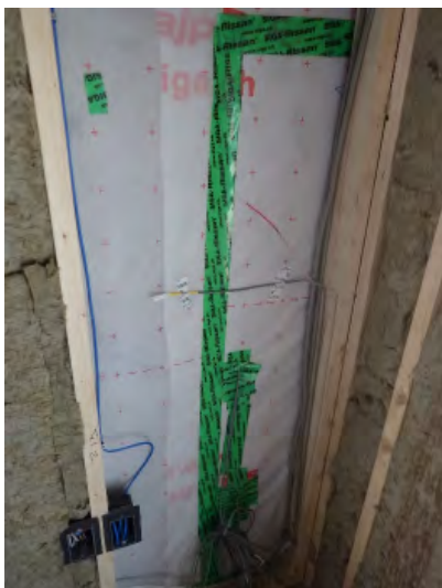
Figure 3-6 – S2 interior relative humidity and thermistor in partial installation (awaiting insulation).
