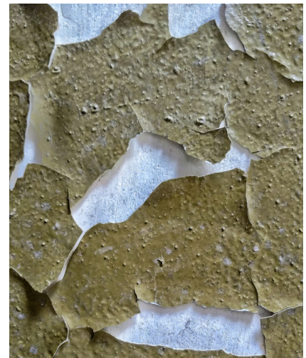
Paint peeling from a metal flashing: Good quality factory-finished metals have better endurance than this site-painted metal flashing.
