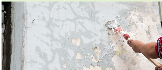
Cleaning and scraping of stucco walls before applying new paint.
