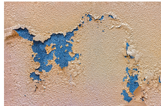
Coatings will not remain adhered if water is permitted to absorb into the material it is intended to protect. As shown here, coating can peel when this occurs.
