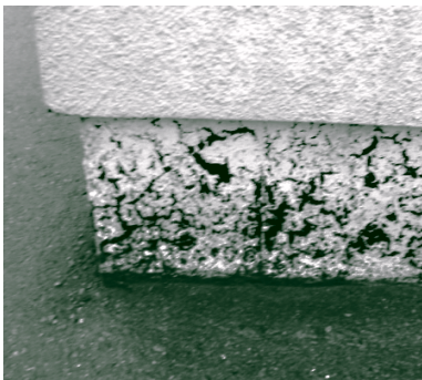
Some coatings such as this acrylic stucco coating over tar-based damp-proofing are incompatible, resulting in a cosmetic detractor instead of providing protection.
