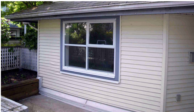
Vinyl siding is made from plastic (mostly polyvinyl chloride) and is intended to simulate the appearance of wood siding. A variety of colours and textures are available. Maintenance is focused on cleaning.
