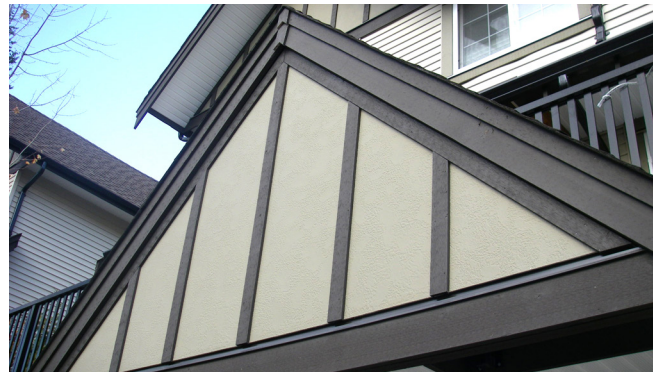
Fibre cement board is a composite material comprised of wood fibre, sand, and cement. The product is painted, and is available as a panel, siding or shingles. Maintenance and renewal activities are focused on cleaning and repainting.
