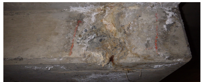
Spalling concrete
