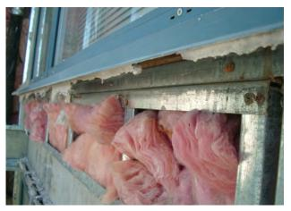
Corroded screws in stud wall beneath window
