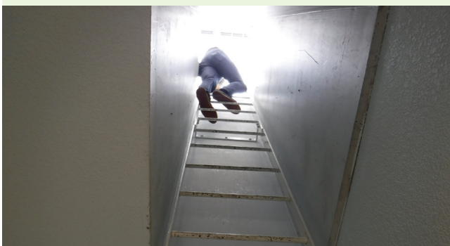
Figure 6: Roof access via hatch.
