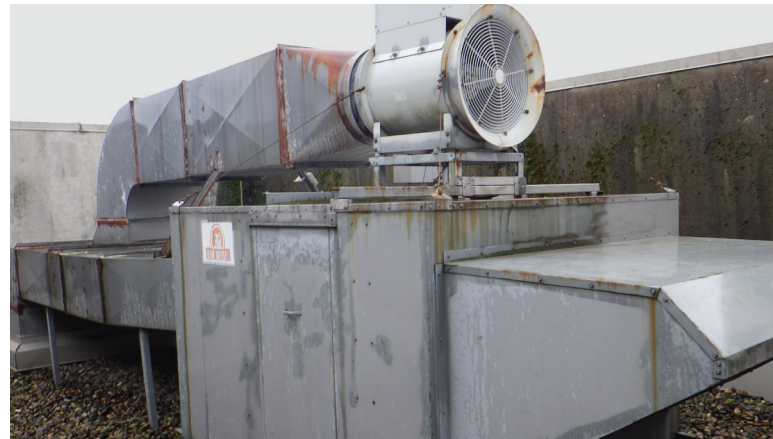
Figure 1: MUA with fire exhaust.
