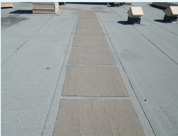
Figure 5: Sacrificial layer of waterproof membrane leading from the roof hatch to the MUA.
