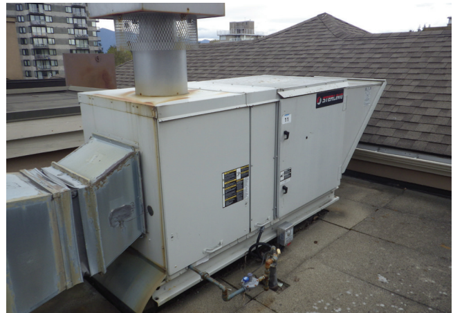
Figure 3: Gas-fired MUA, including the electrical connections.
