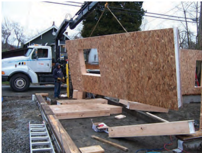
Installation of structural insulated panels (SIPs) at a laneway home construction site. Source and image credit: Lanefab homes.
