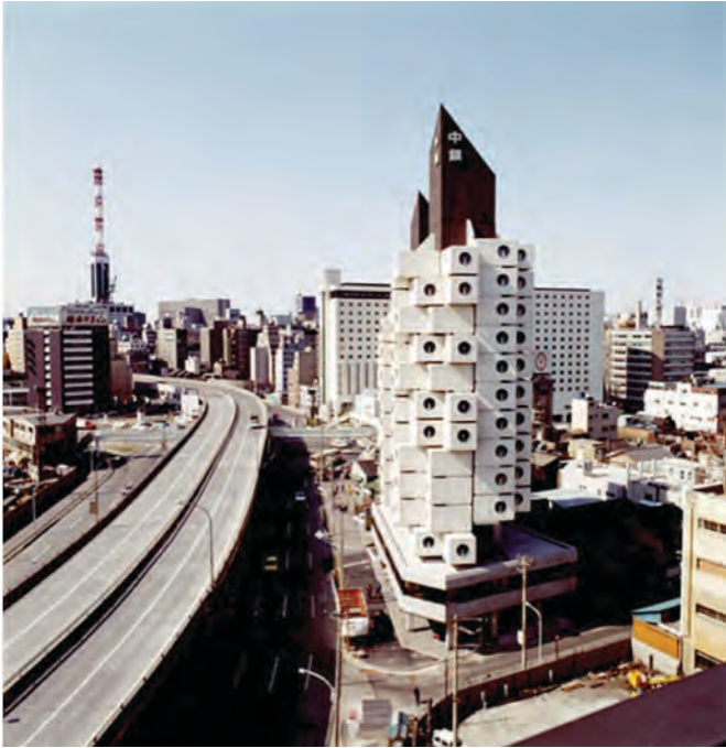
Nagakin Capsule Tower in Toyko Japan was built in 1972 with modular components, and is comprised of many apartment capsules. Source and Image credit: Megan Sveiven, February 9, 2011.
