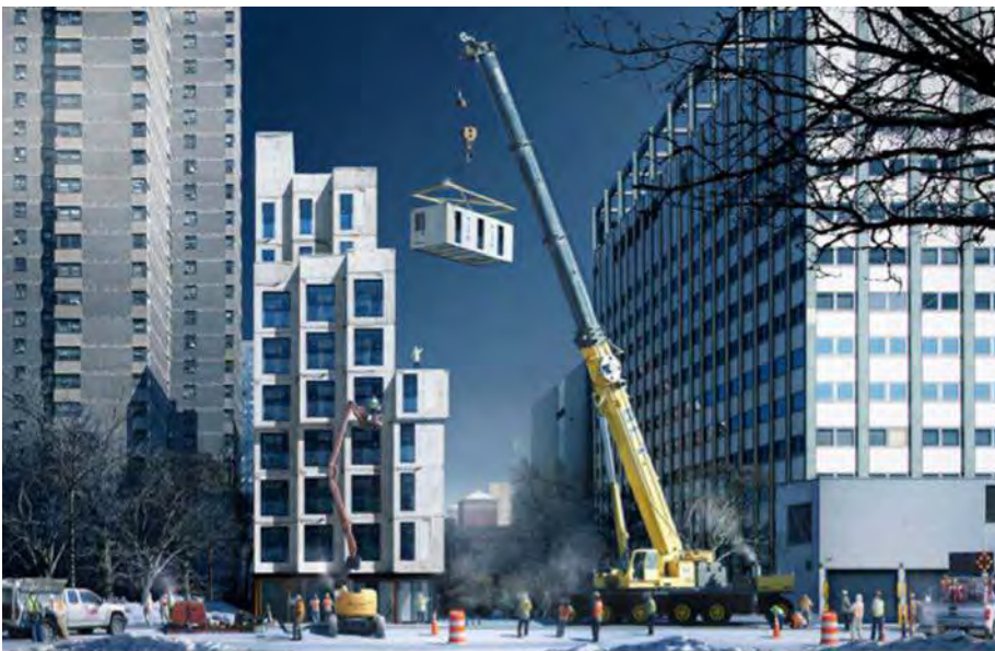
Rendering of installation of modules at My Micro New York pilot project site. Source and image credit: nArchitects.
