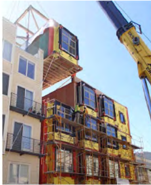
Installation of modules for micro-apartment building at 38 Harriet Street, San Francisco. Source and image file: Panoramic Interests and Zeta communities.
