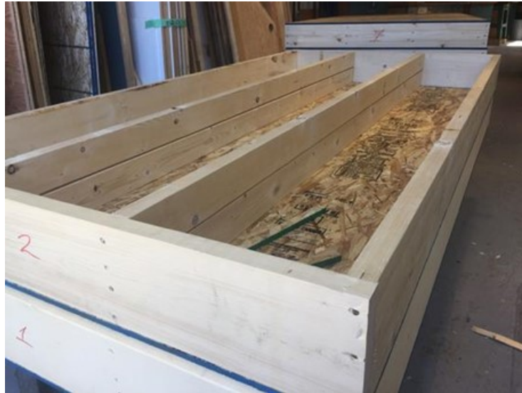
Figure 119. A double-stud wall with a 6 mm gap between the two rows of studs
