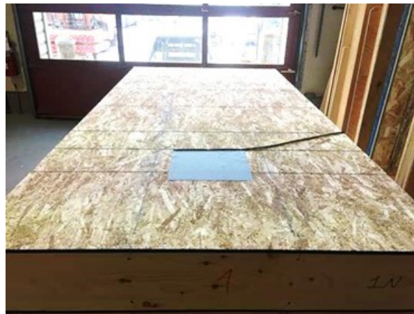
Figure 120. A paper towel together with a plastic tube installed on the exterior surface of the OSB sheathing for injecting water in the future
