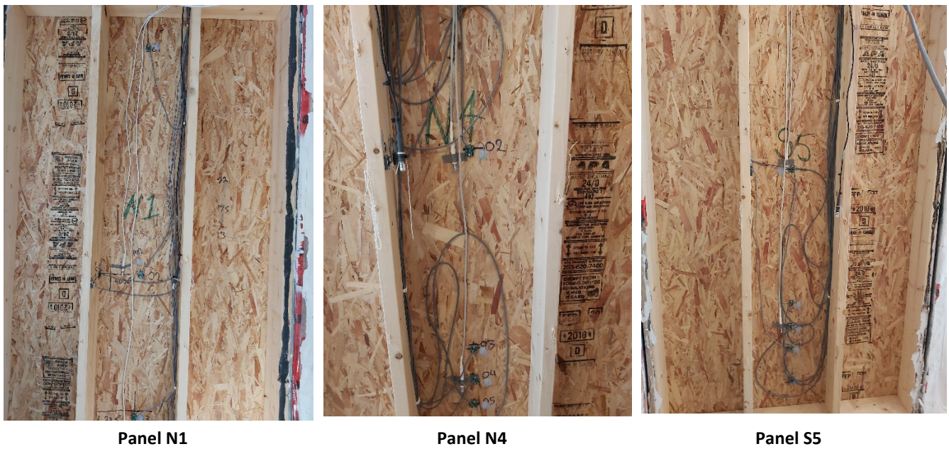
Figure 117. Visual condition of OSB sheathing of selected wall panels at the completion of testing in July 2020
