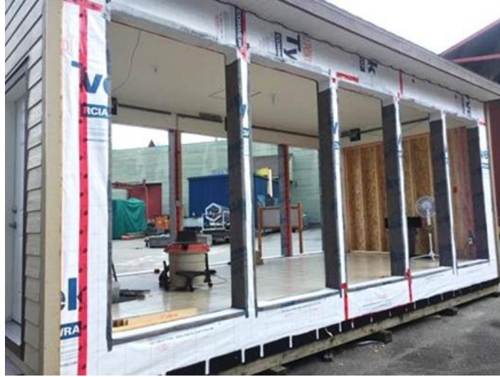
Figure 121. The perimeter of each wall opening pre-sealed with membranes, with gasket installed at the bottom
