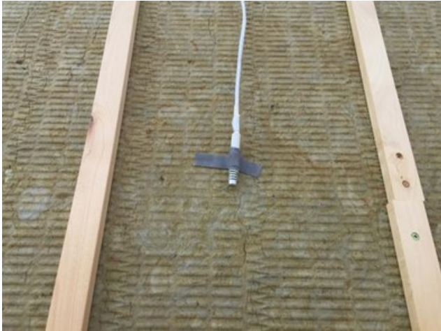
Figure 122. An RH/T sensor installed in the rainscreen cavity, being exterior to the exterior stone wool insulation
