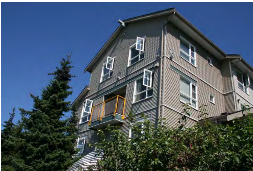
Figure A12. Location of rain gauges installed on Bldg. 4
