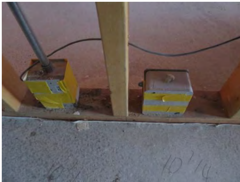
Figure 1 Displacement sensor boxes sitting on the bottom plate of an interior partition wall
