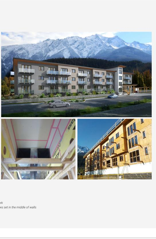
**Top** Orion, Vidorra Developments Bottom Left Soffit insulation with simple ventilation ductwork Bottom Right Wood frame structure with triple-pane windows set in the middle of walls
