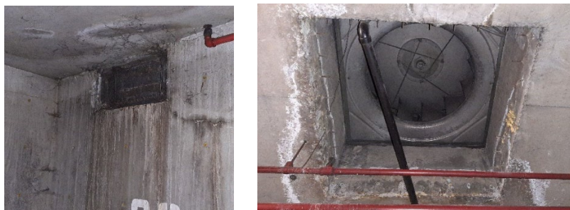
Figure 74. Parkade makeup air and exhaust fan
