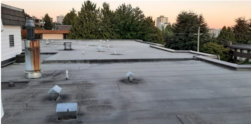
Figure 72. Rooftop kitchen and bathroom vents, boiler exhaust, and corridor ventilation unit
