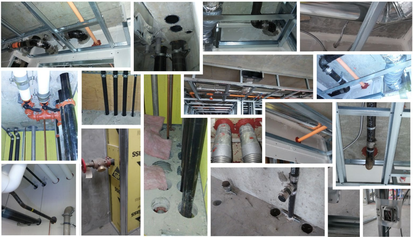
Figure 55. Photos of compartmentalization air leakages, with a few of them being sealed with red fire-rated sealant
