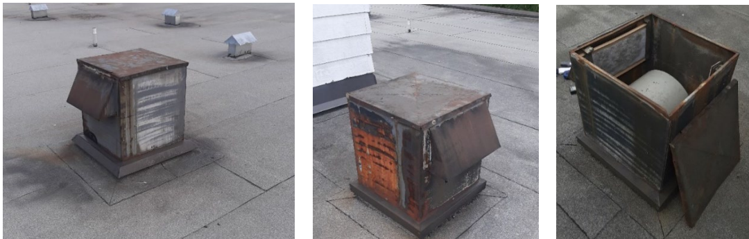
Figure 73. Two rooftop ventilation units for the entire building
